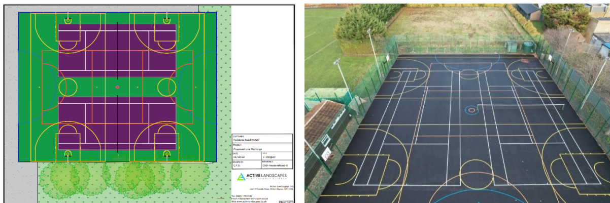
Haydons Road Recreation Ground MUSA prior to colour coating and line marking
